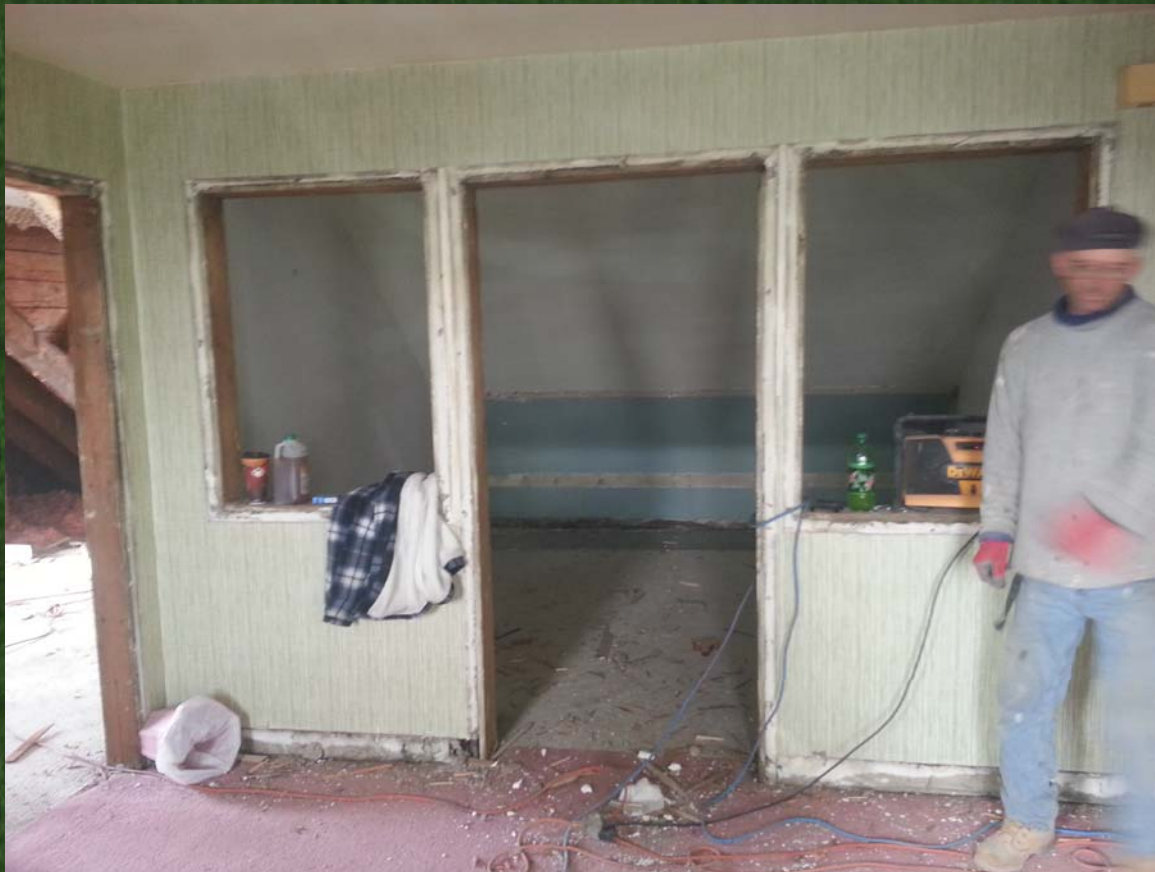
Future Third Floor Study Room
